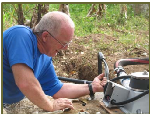
John Whited connecting the turbine
