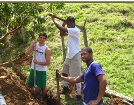
Digging a ditch for the piping
