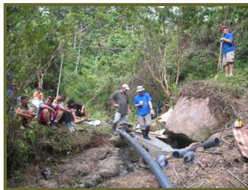
Manuel and John and the team working on the intake
